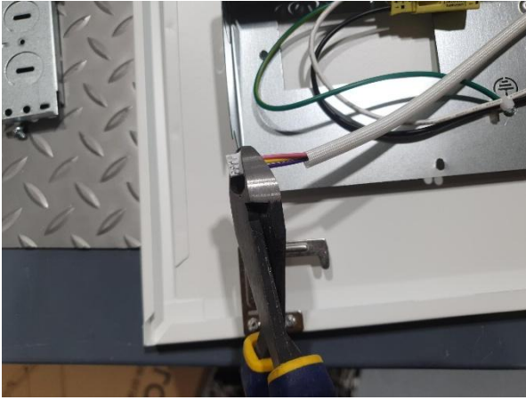
3. Cute the three wires
